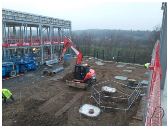
Courtyard – Canopy Bases
