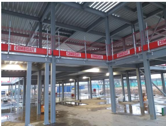
Ground Floor Main Hall - Zone 2
