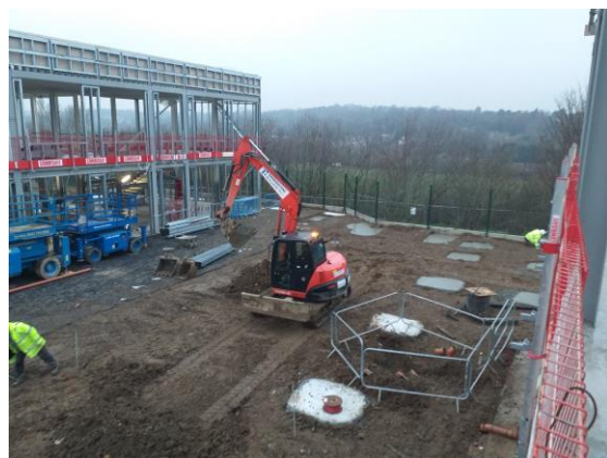
Courtyard – Canopy Bases
