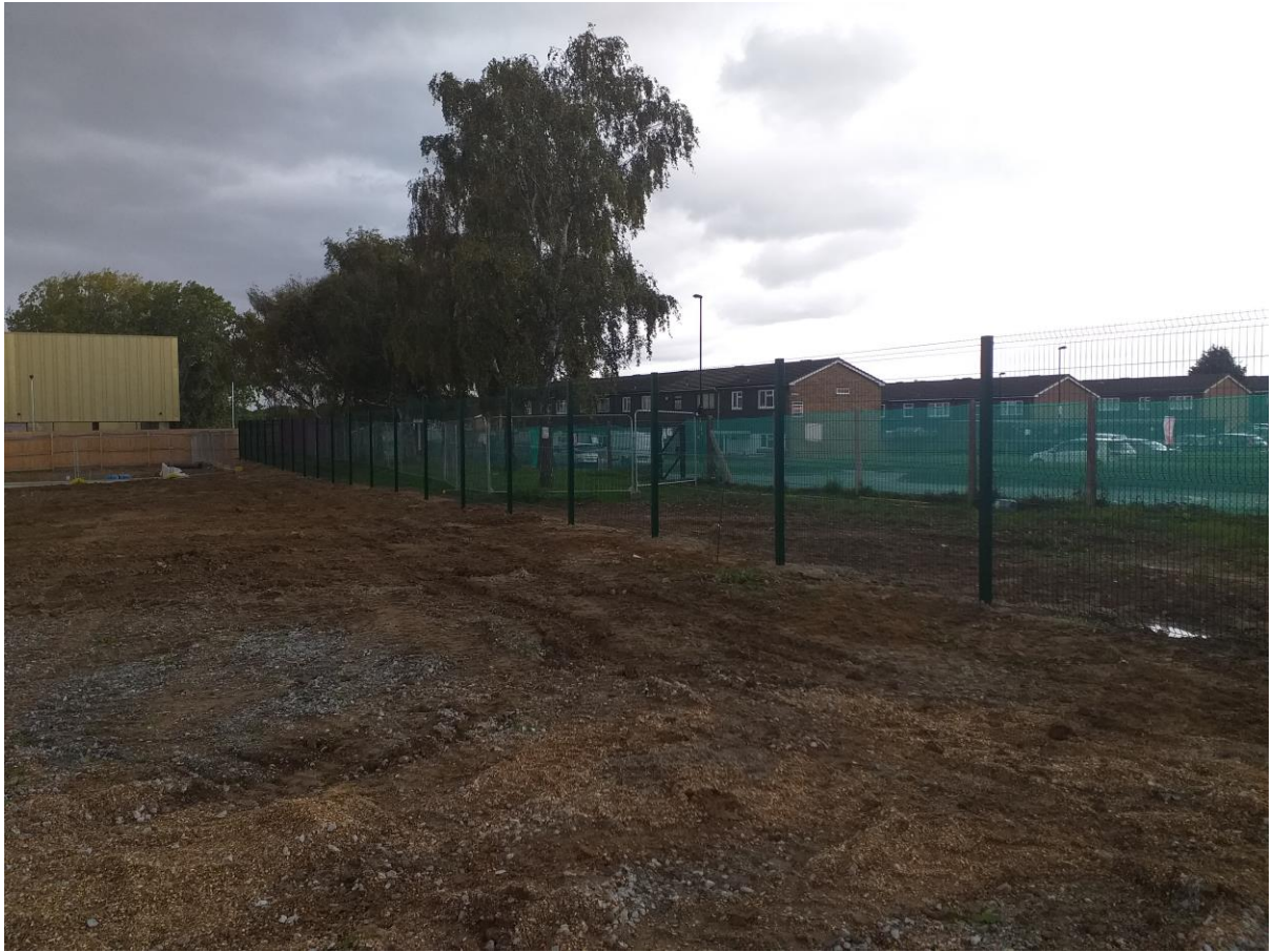
New Perimeter Fence
