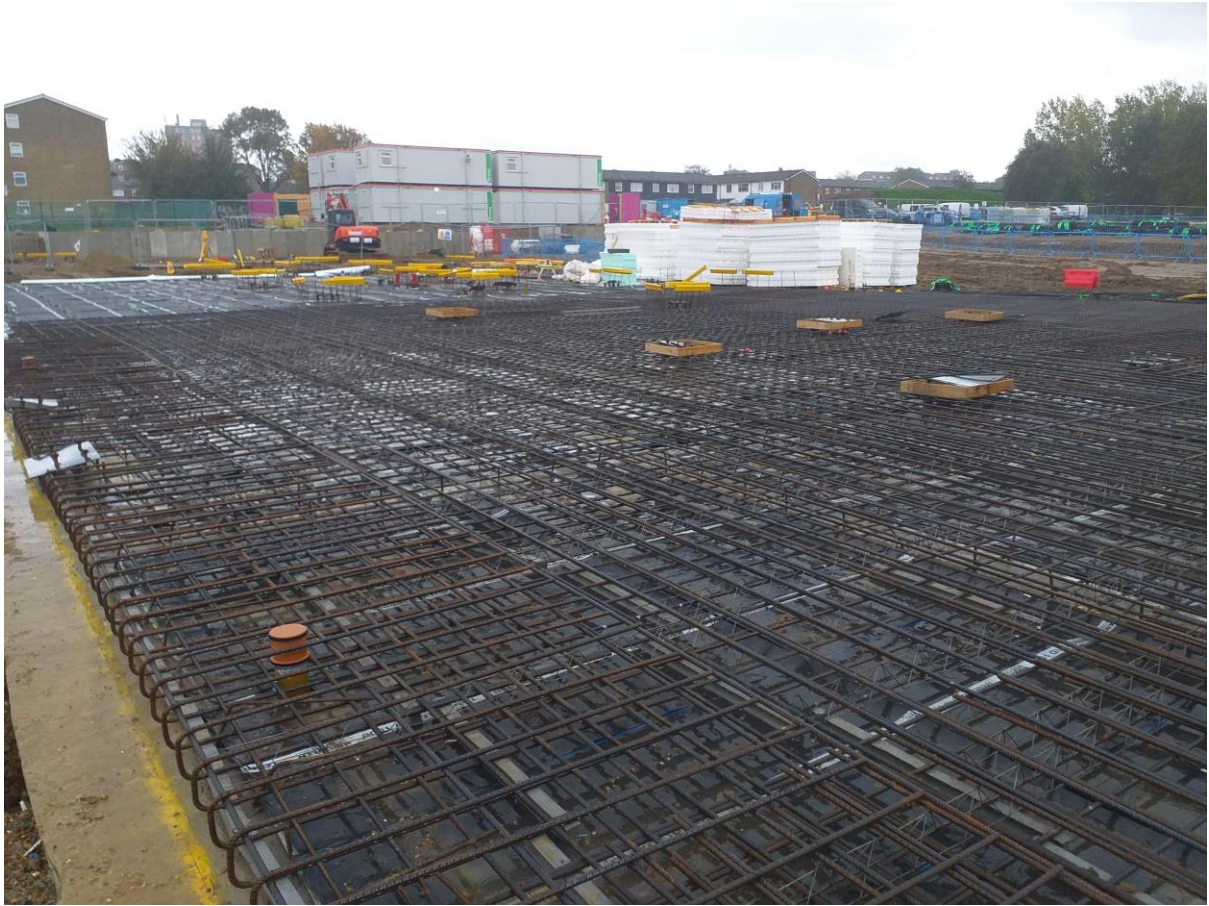
Ground Floor Slab – Zone 1
