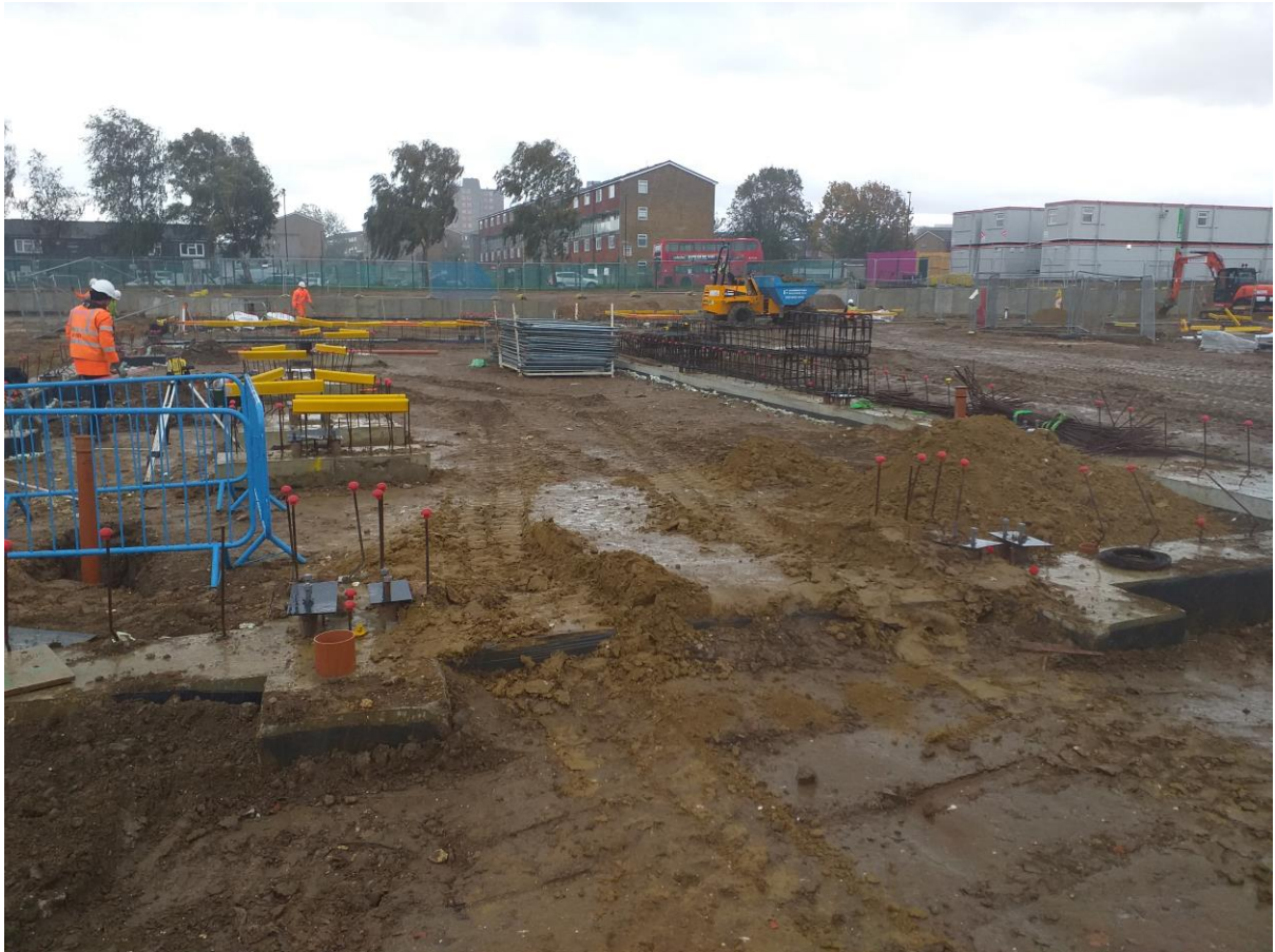
Pilecaps Groundbeams and Drainage
