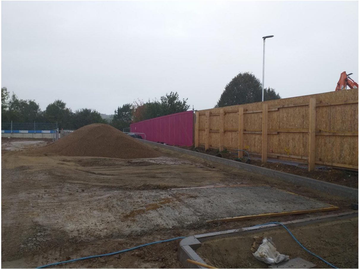
East Car Park Kerbs
