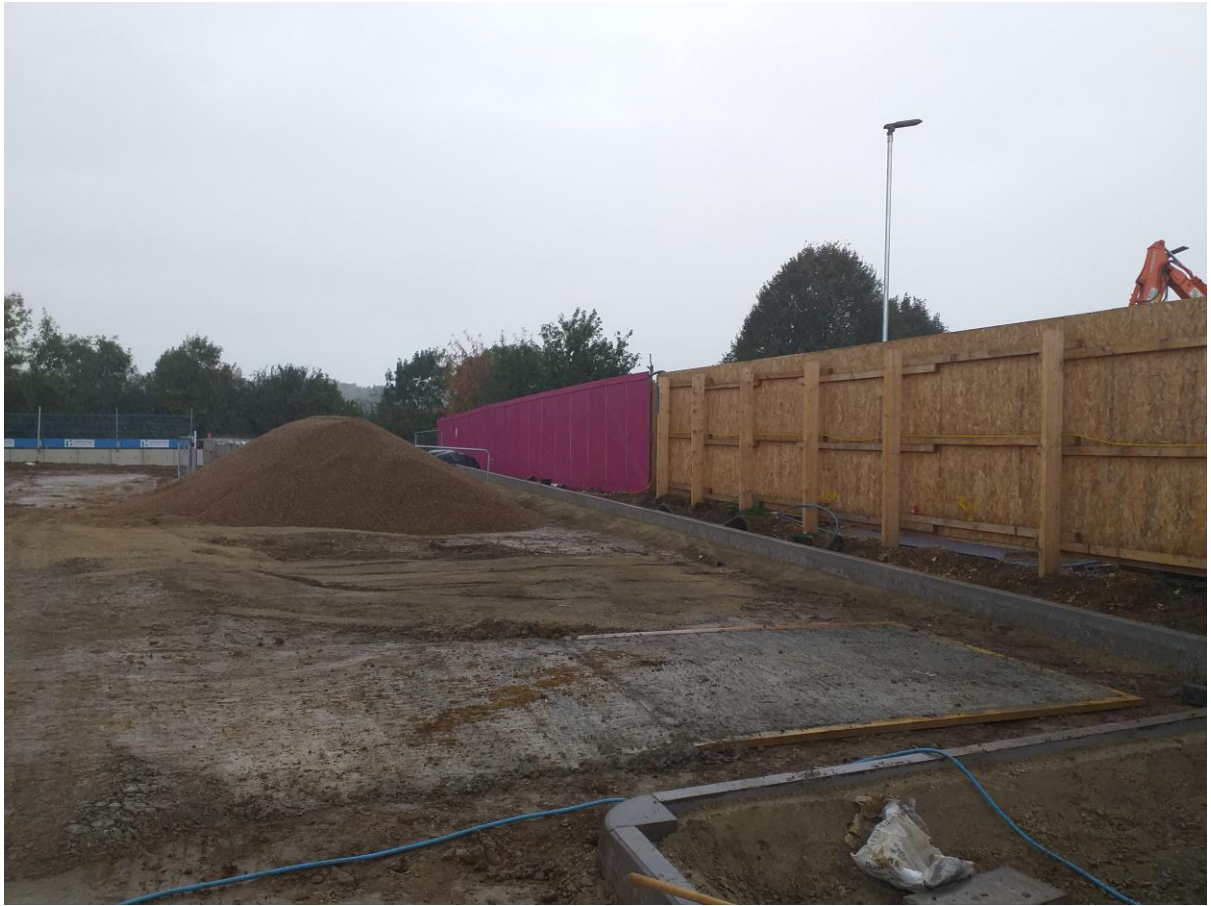
East Car Park Kerbs
