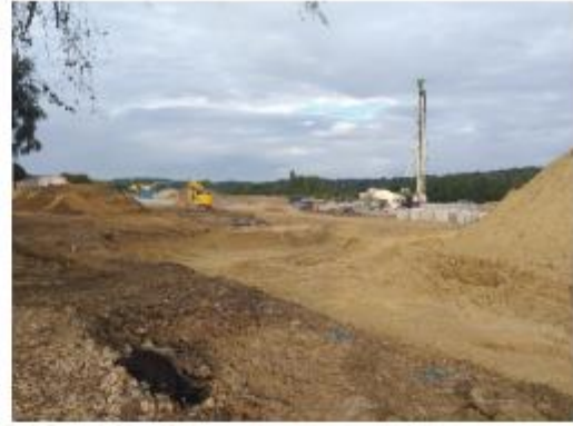
Excavation for Retaining Wall
