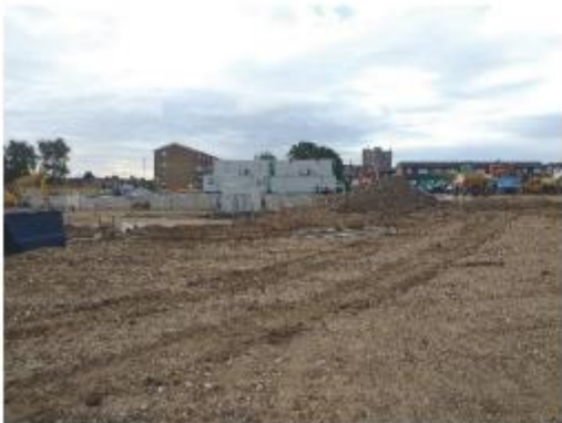
Retaining Wall and Site Office
